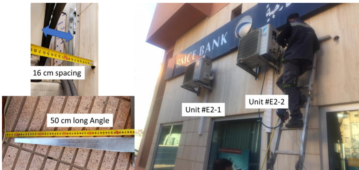
(b) New RAC Outdoor Units Installation
